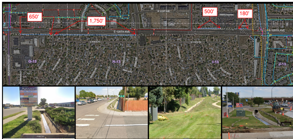
Figure 1 – New Union Ditch Existing Concrete Channel
