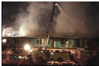
Caption: “Thornton firefighters spray water onto the Hacienda Hotel, in hopes of extinguishing the blaze.”
