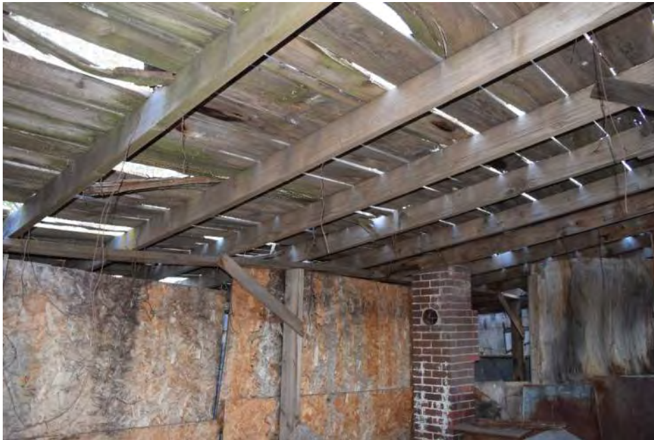
Figure 5. Readily visible structural members of Outbuilding #1.
