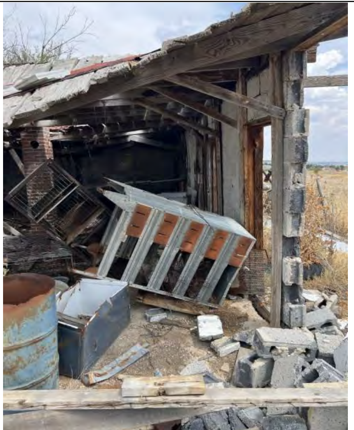
Description: Structure 5, ACM Roofing Tar & CMU Patch Tar 7/15/24 Inspection
