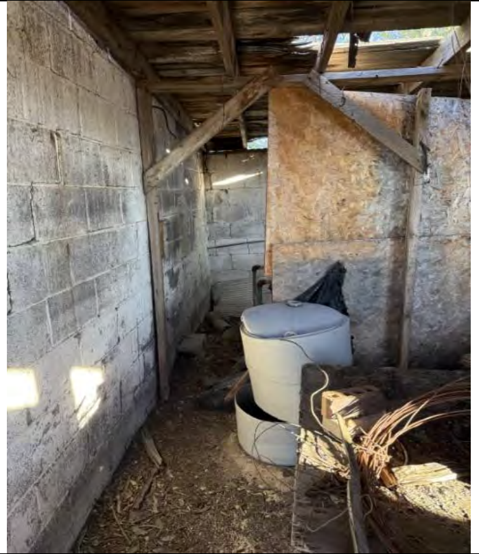
Description: Structure 7, north-center "tack" room interior
