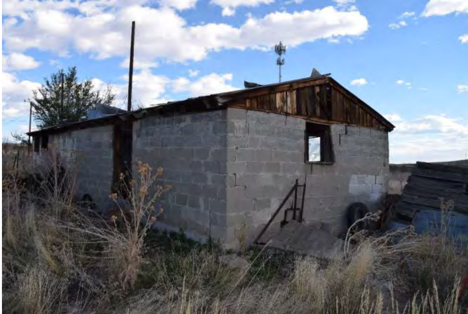
Figure 8. Overall view of Outbuilding #2 from the southwest corner.
