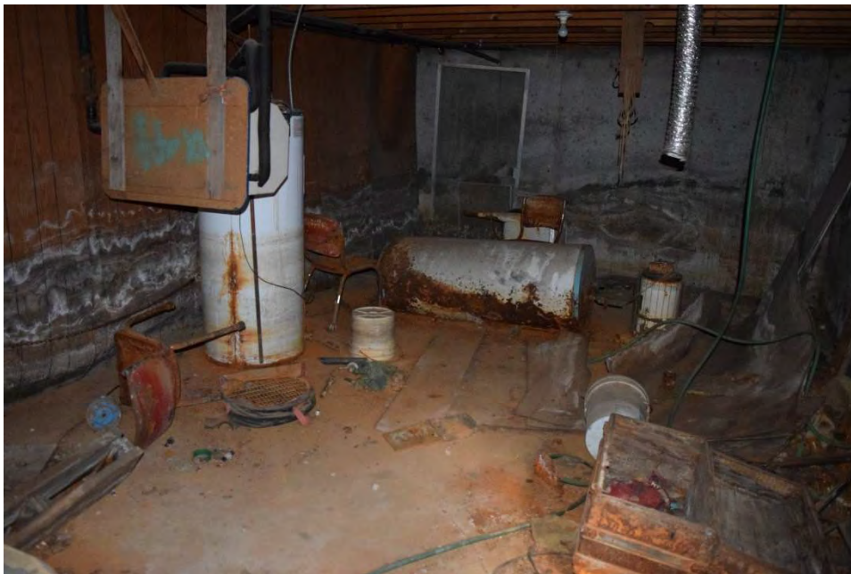
Figure 5. Underground basement below the west half of the Original Farmhouse.
