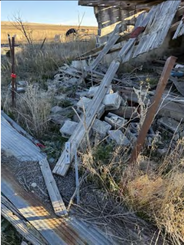
Description: Structure 5 10/28/25 Inspection
