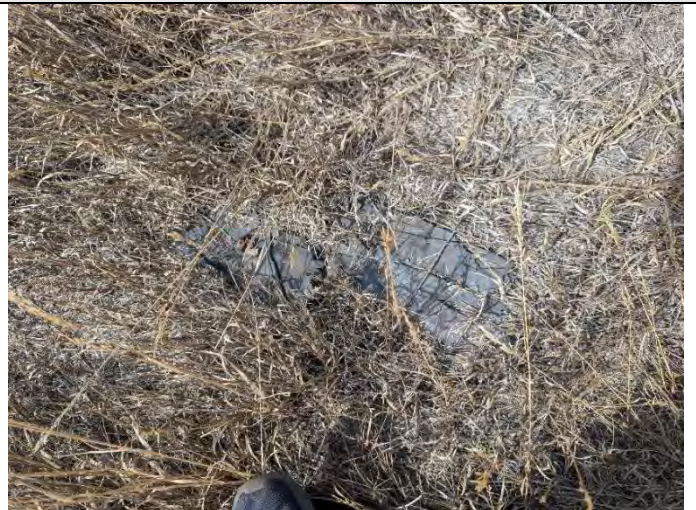
Description: Structure 5 Debris 9/9/25 Inspection
