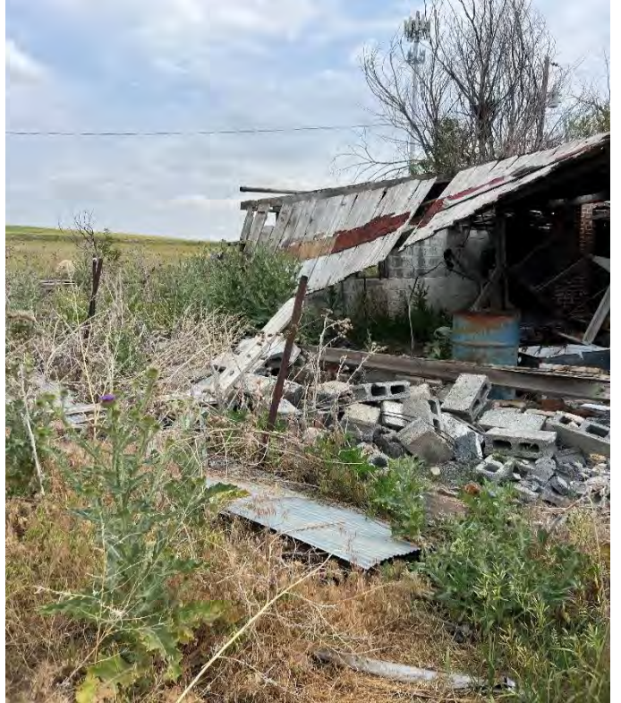
Description: Structure 5, ACM Roofing Tar & CMU Patch Tar 7/15/24 Inspection
