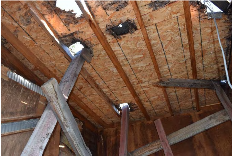
Figure 10. Penetrations through roof structure of the Well House .
