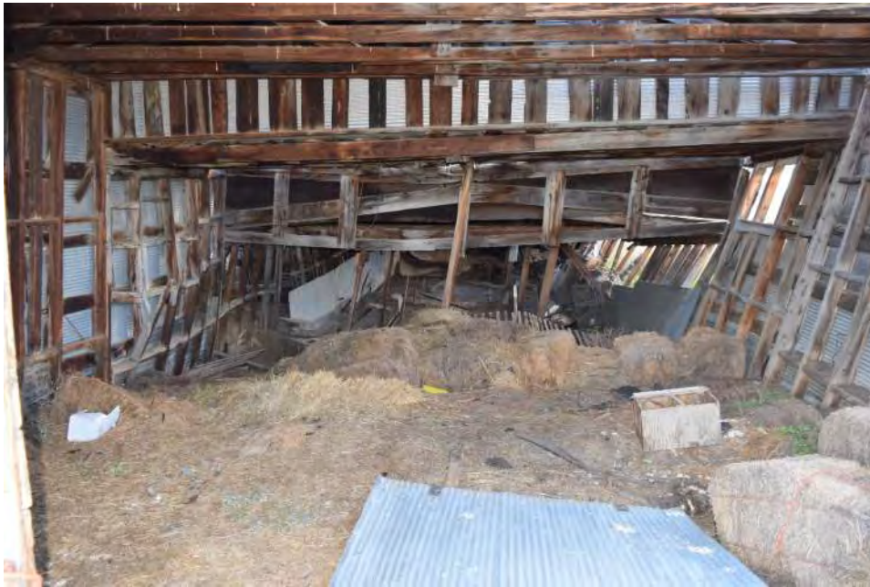
Figure 15. Structural members of the Hen House from the east side.
