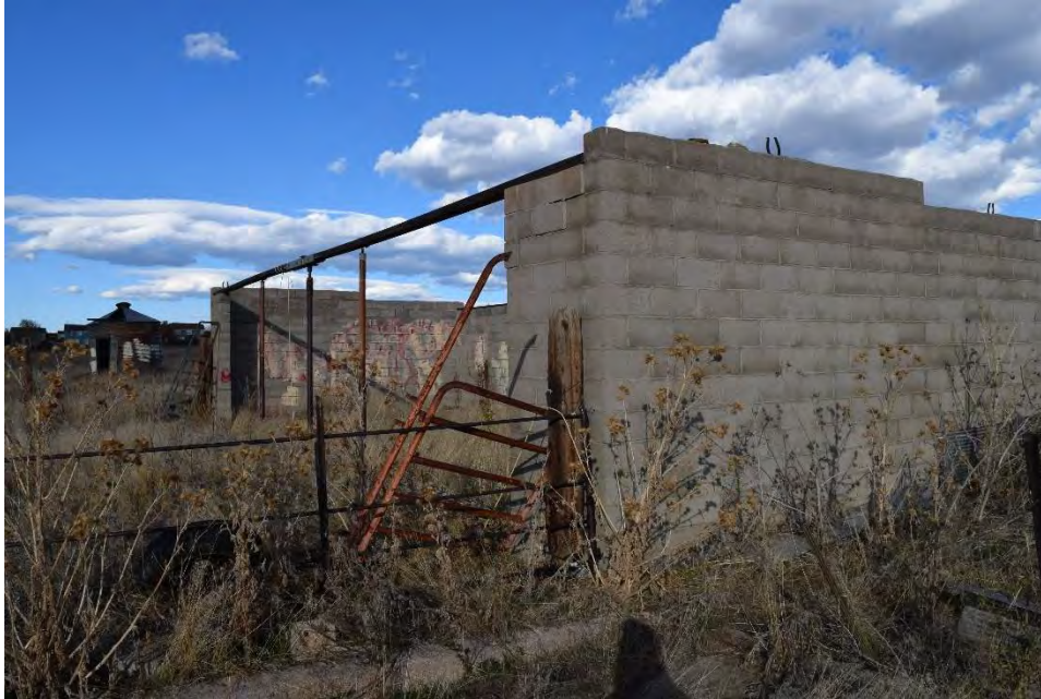
Figure 18. Overall view of the CMU Wall Enclosure from the southeast corner.
