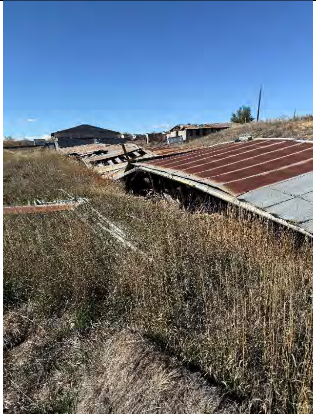
Description: Structure 6 10/28/25 Inspection
