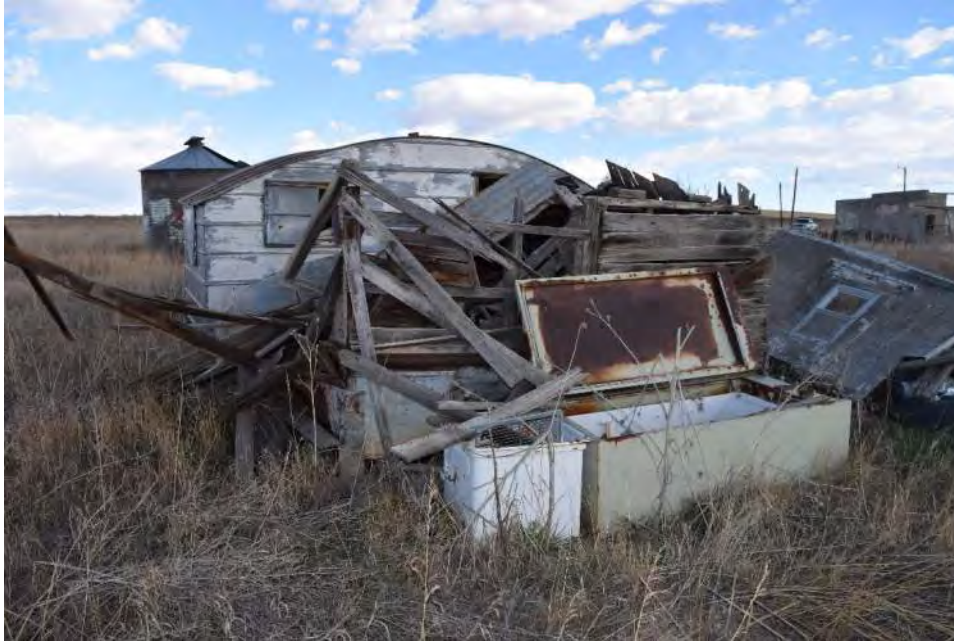
Figure 12. Overall view of Outbuilding #3 from the southwest corner.
