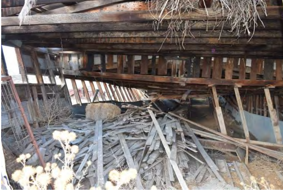
Figure 16. Structural members of the Hen House from the west side.
