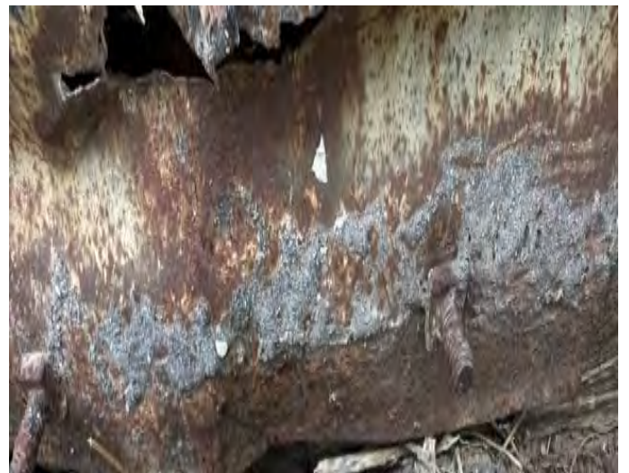
Description: Structure 10, ACM Tar Sealant 7/15/24 Inspection
