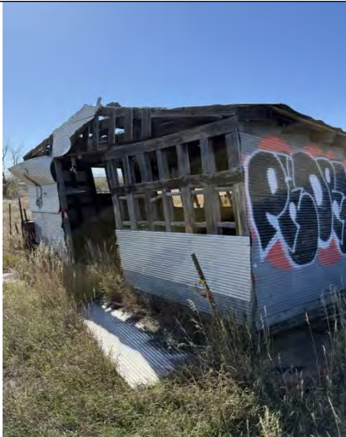
Description: Structure 6 west end
