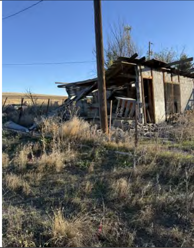
Description: Structure 5, west side
