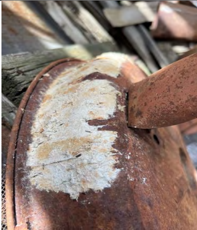
Description: Structure 9, ACM Paper 7/15/24 Inspection
