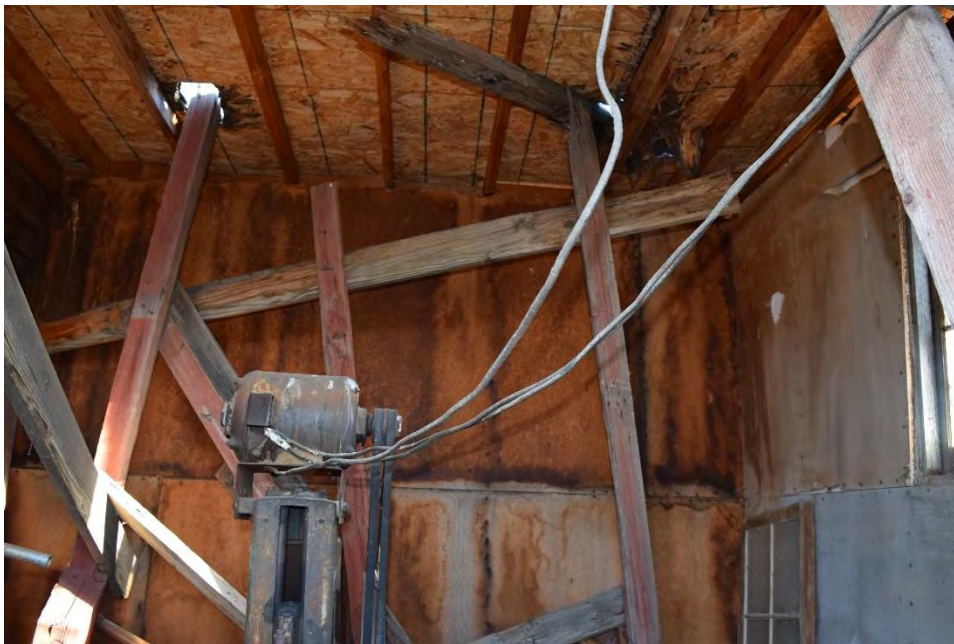
Figure 9. Interior view of the structural members of the Well House.
