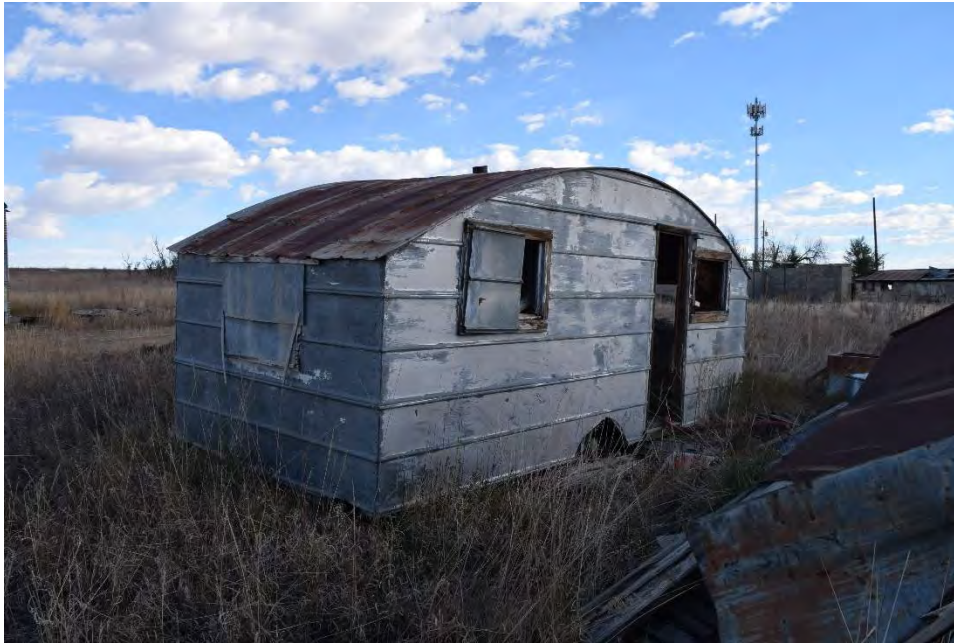
Figure 20. Overall view of the Camper from the southwest corner.
