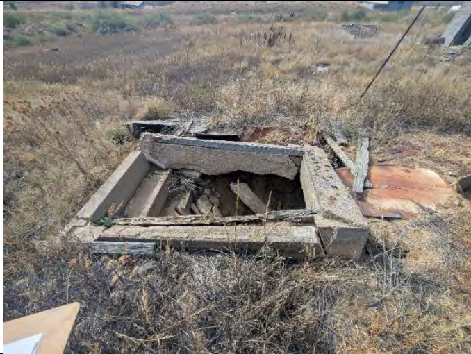
Description: Structure 3 9/9/25 Inspection
