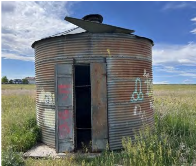
Description: Structure 10 7/15/24 Inspection
