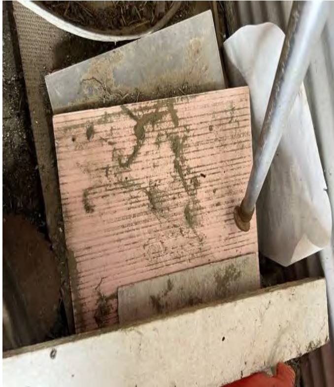
Description: Structure 3, ACM Cementitious Siding 7/15/24 Inspection
