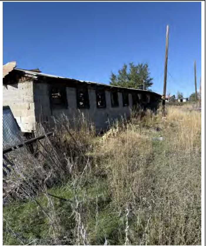
Description: Structure 7, west side
