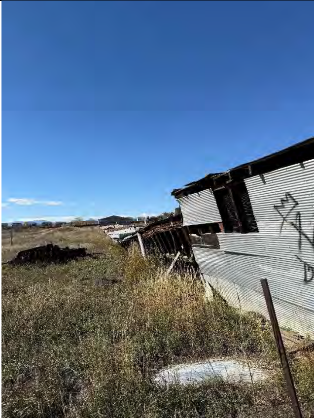
Description: Structure 6 10/28/25 Inspection
