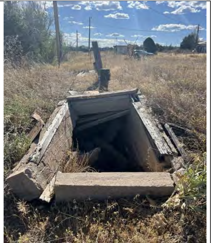
Description: Structure 3 East Entry 7/15/24 Inspection
