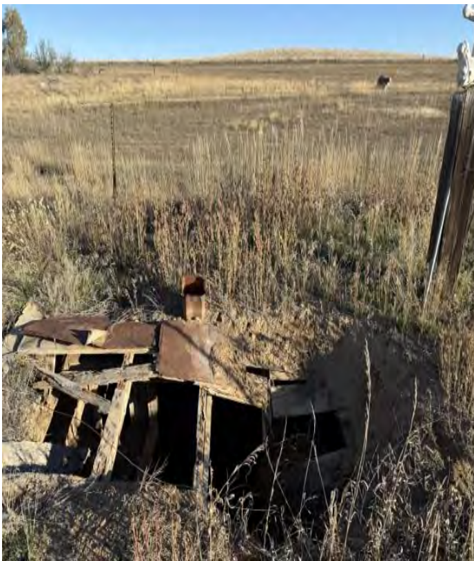
Description: Structure 4 10/28/25 Inspection
