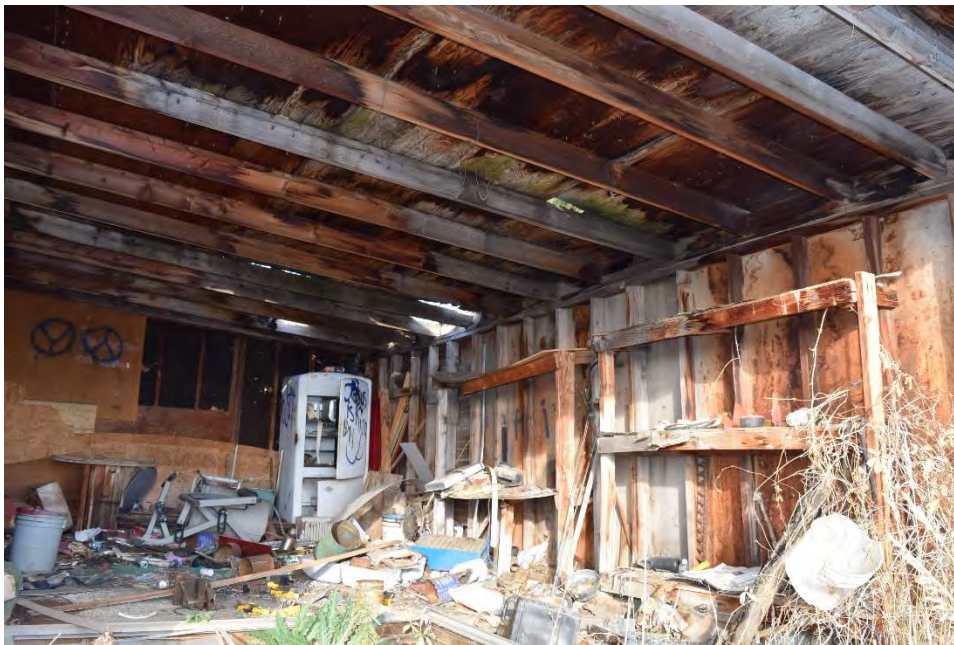
Figure 13. Structural members of the partially enclosed area of the Garage.
