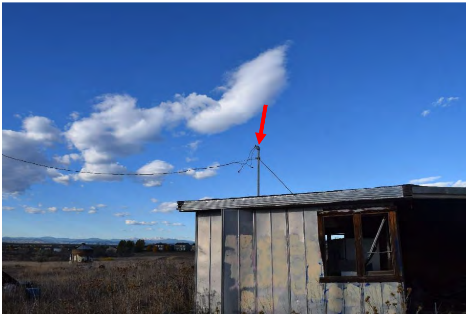
Figure 15. Wires entering the Garage in the southeast corner.
