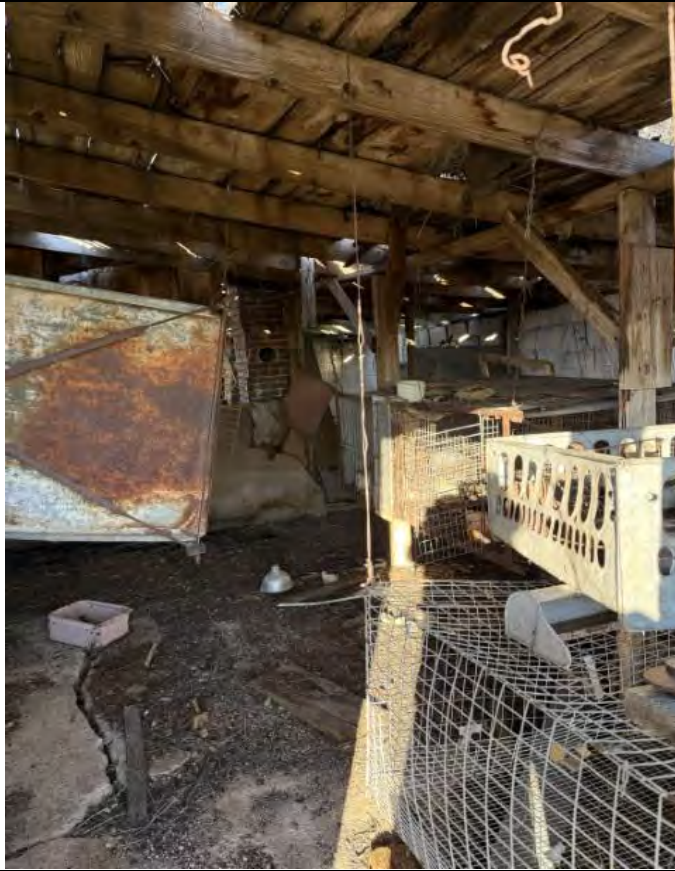
Description: Structure 5, east side
