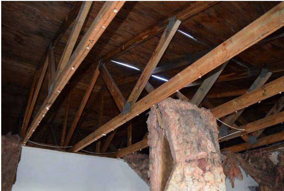
Figure 3. Wood roof trusses in the west half of the Original Farmhouse.
