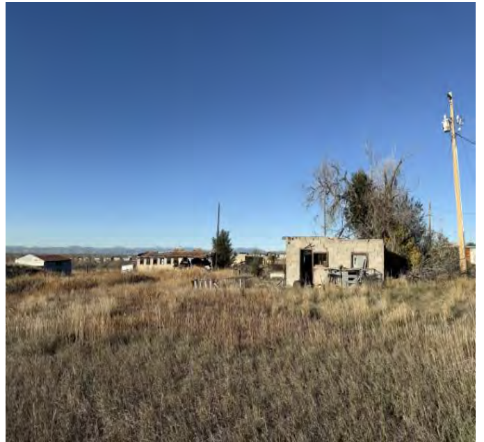
Description: Overview of the Buildings onsite looking NW
