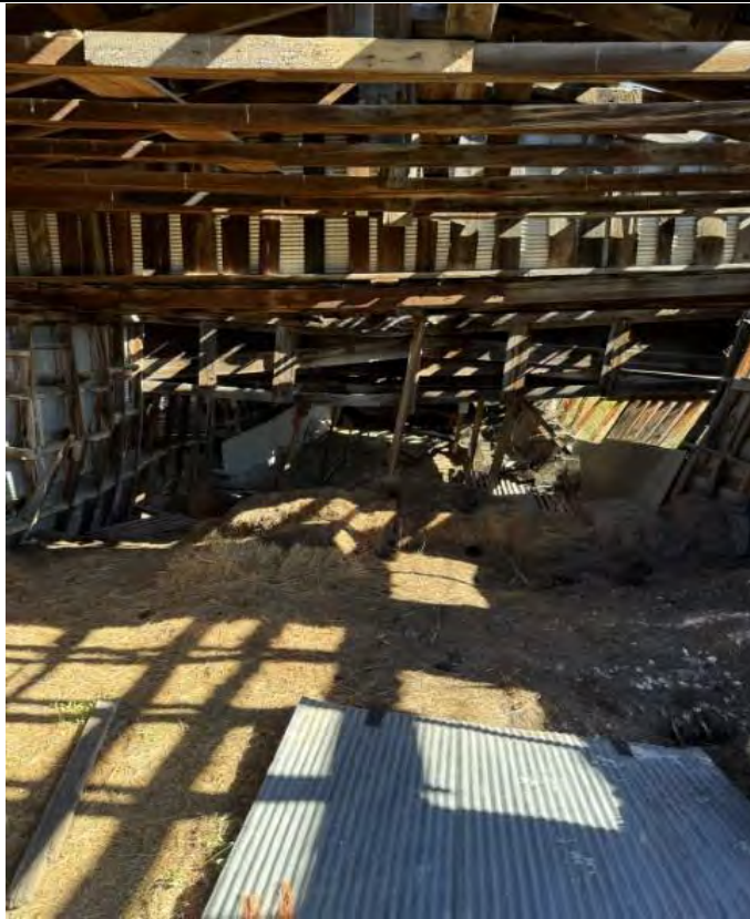
Description: Structure 6, west end of inside
