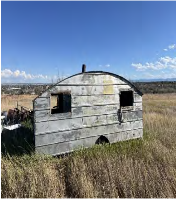
Description: Structure 11 7/15/24 Inspection
