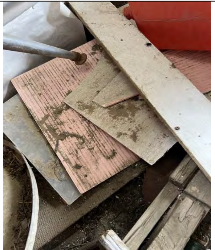
Description: Structure 3, ACM Cementitious Siding 7/15/24 Inspection
