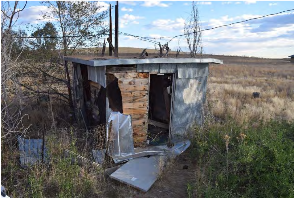
Figure 8. Overall view of the Well House from the southeast corner.
