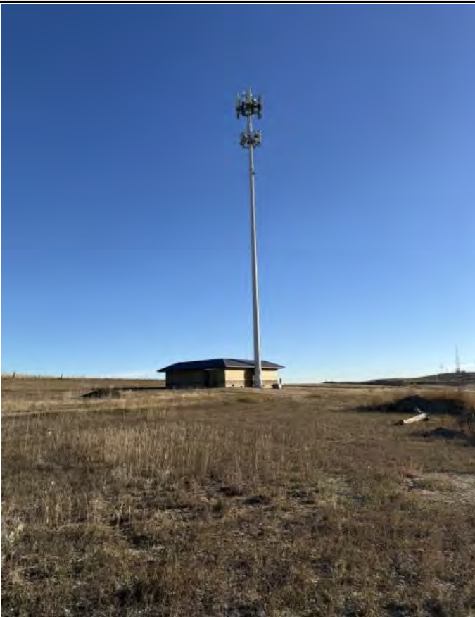
Description: Telecommunications Radio Tower
