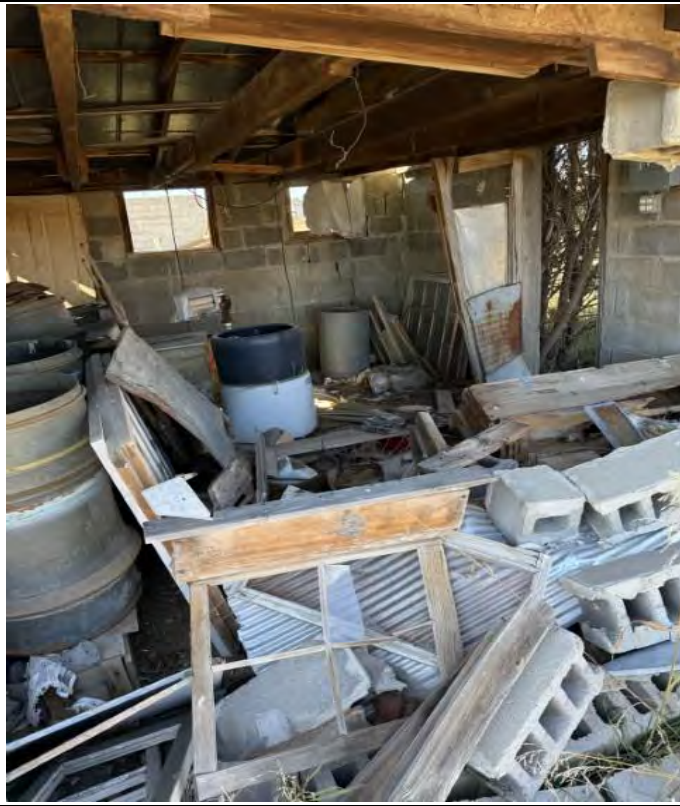
Description: Structure 7, north "tack" room interior
