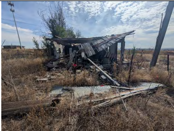
Description: Structure 5 9/9/25 Inspection
