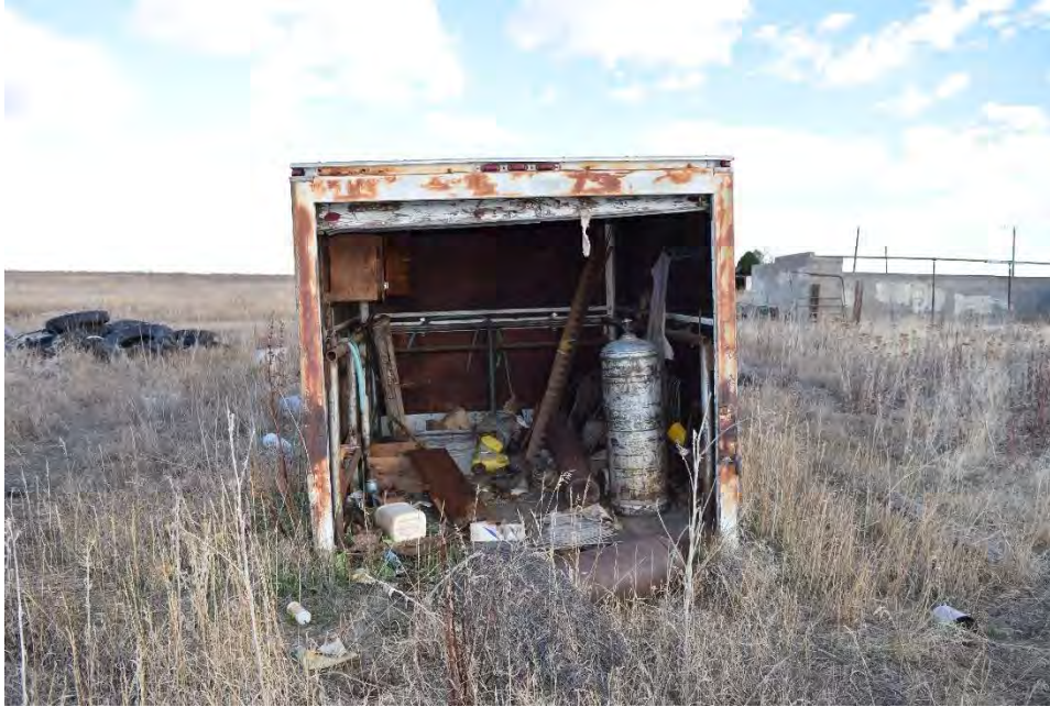
Figure 22. Overall view of the Trailer from the south.
