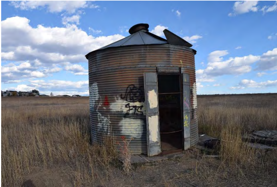
Figure 16. Overall view of the Silo from the southeast corner.
