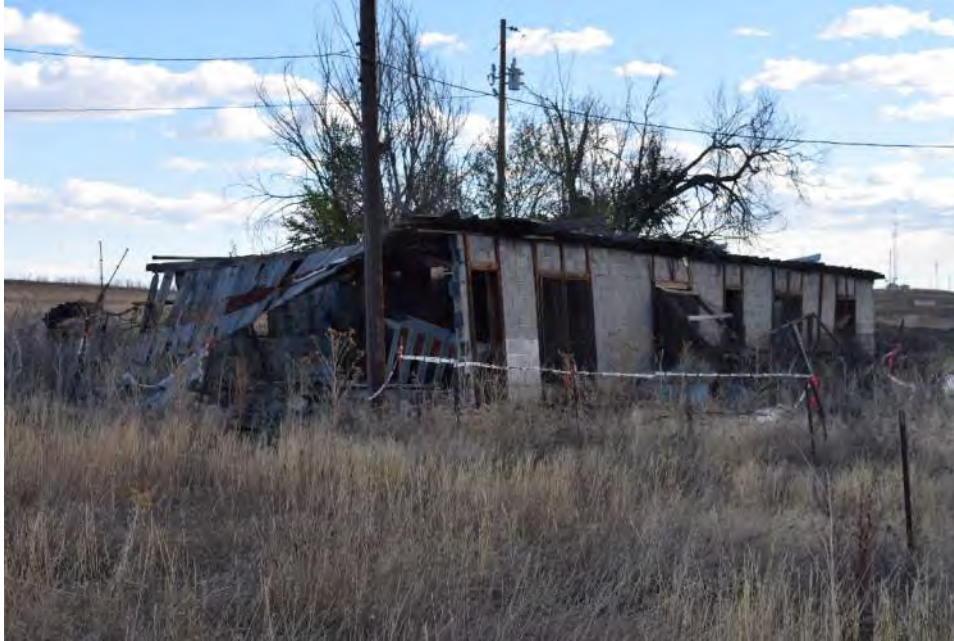
Figure 4. Overall view of Outbuilding #1 from the southwest corner.
