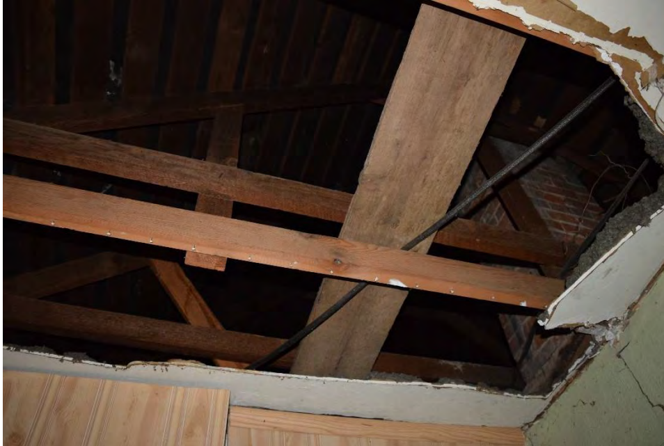
Figure 4. Wood roof trusses in the east half of the Original Farmhouse.
