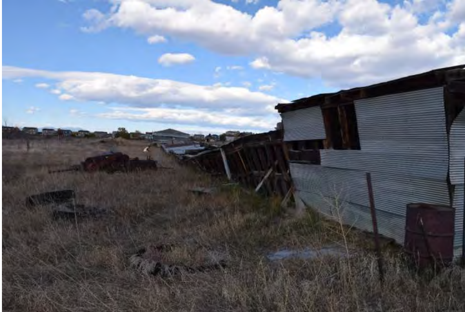
Figure 14. Overall view of the Hen House from the southeast corner.
