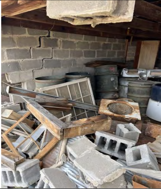
Description: Structure 7, ACM Window Glazing 7/15/24 Inspection
