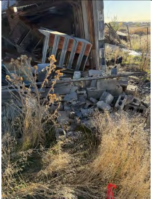
Description: Structure 5 10/28/25 Inspection
