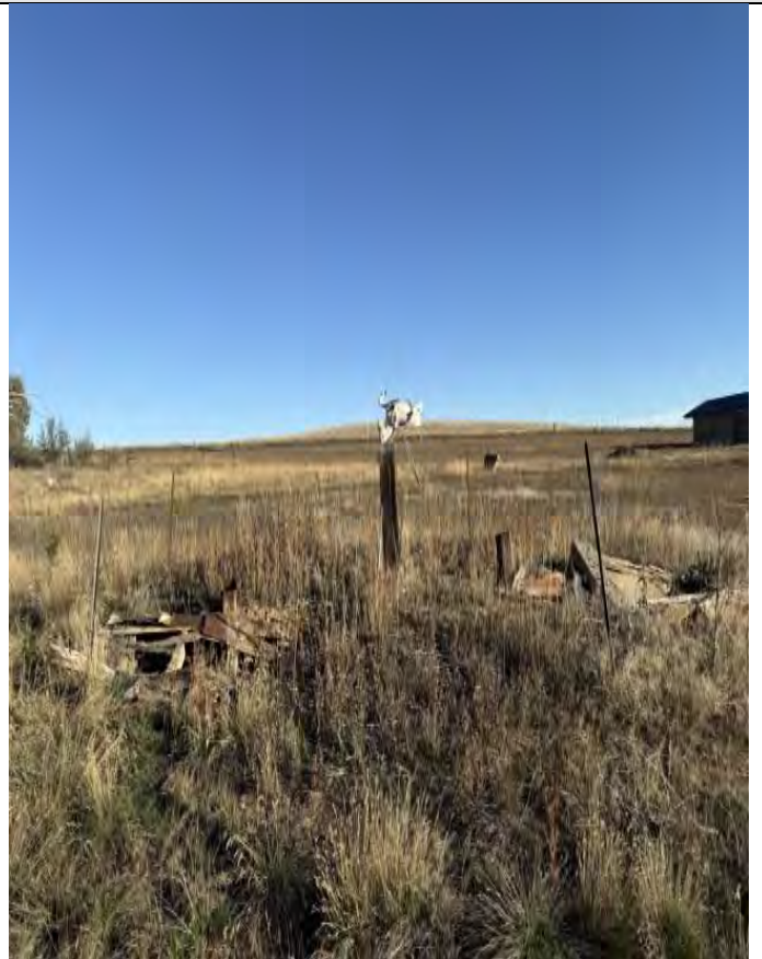
Description: Structure 3, vents and roof of the sub-terranean structure
