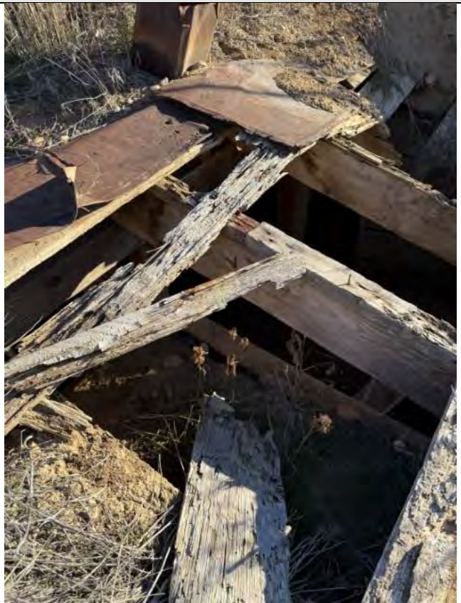
Description: Structure 4 10/28/25 Inspection
