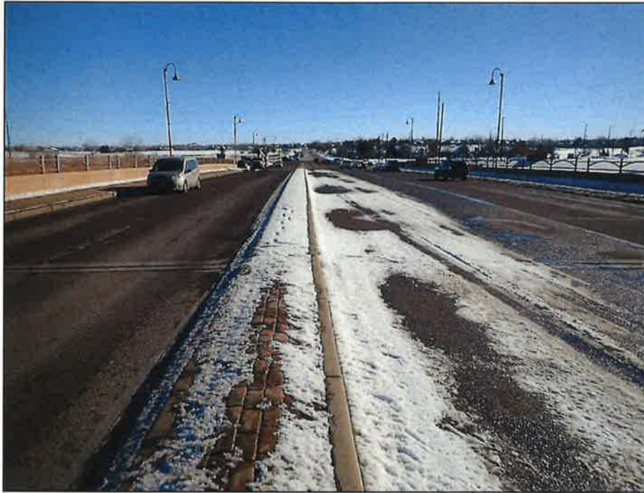
Roadway, Looking East
