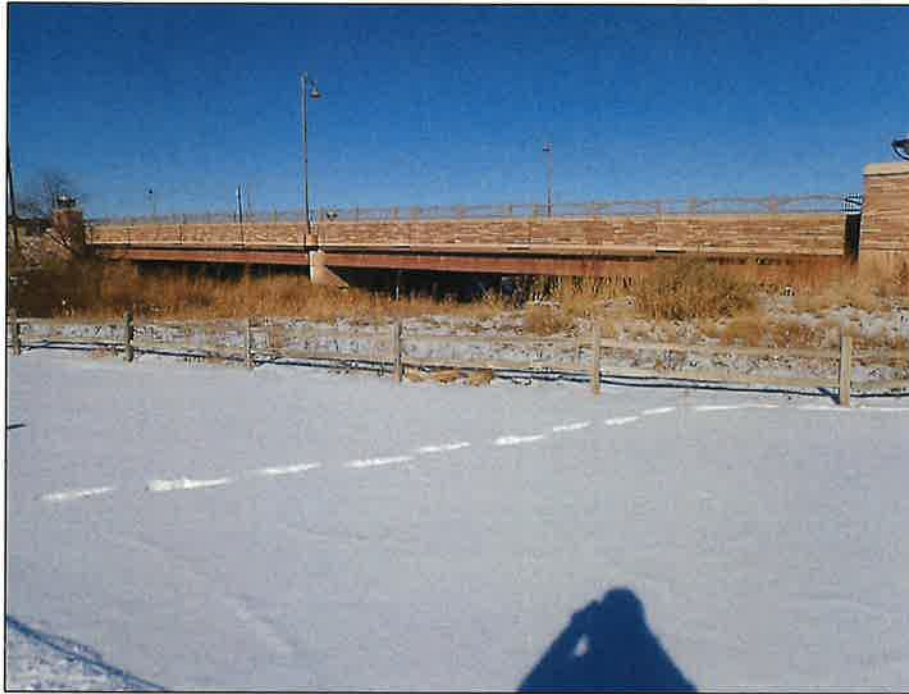
Elevation, Looking North
