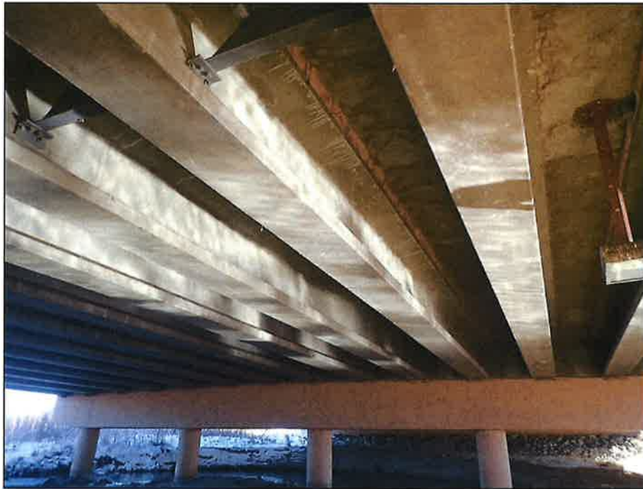
Superstructure, Looking West
